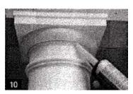
**10.** Apply a paintable silicone caulking between the capital and the shaft. (**NOTE: Not all silicone caulking is paintable.**)
