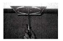
NOTE: If using ER Cap Flashing Kit it is important to center and fasten the flashing to soffit using #10 wood screw (provided) prior to beginning step one. The screw should be used as the center point of soffit to drop plumb bob.
