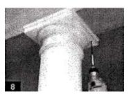
8. Slide the capital into place, pre-drill through the capital, and secure the capital to the soffit above using rust resistant screws. Use automotive body filler to cover the screw heads.
