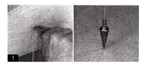
1. Drop a plumb bob from the center of the soffit to determine the column's center point on the floor. Mark this point for reference to align the shaft in the proper position.
