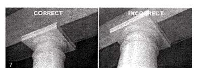
**7.** Remove any bracing and allow the load to bear on the column shaft. Make sure the load is centered over the entire circumference of the column shaft. When in proper position:
