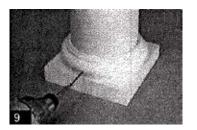
**9.** Pre-drill and attach the base to the column using rust resistant screws. Use automotive body filler to cover the screw heads
