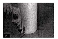
**6.** With the shaft in place, use self tapping masonry screws to secure L-brackets to floor surface. Pre-drill the shaft to receive screws.
