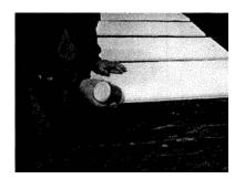
**4.** Apply polyurethane glue to both edges of ONE PANEL only.
