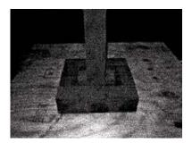
**1.** Install blocking around load bearing support (typically pressure treated post). Blocking should be made from pressure treated wood, and must be the same size as the inside of the pedestal/newel.
