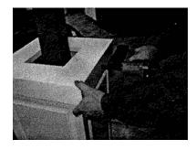
**11.** Apply glue to backs and mitered edges of cap moldings, then assemble to shaft below top platform with screws or pin-nails.
