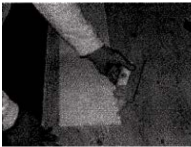
13. Apply adhesive to final panel.
