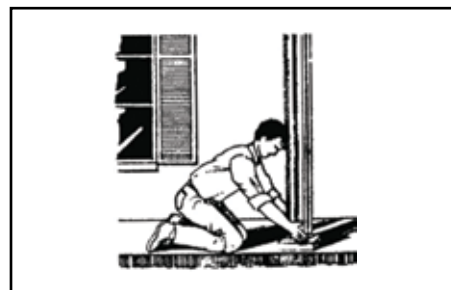
Slide cap and base into place and tighten set screws.
