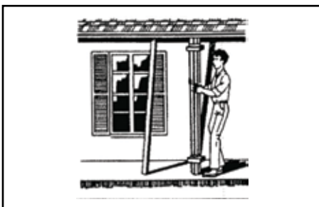
Put cap and base on column. Set in place and plumb with a level. Let weight down on column.
