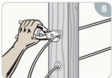
Trim the excess threads on the Threaded Terminal and excess cable behind the Quick-Connect®SS.
