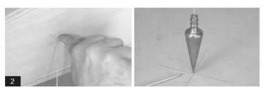
**2**. Drop a plumb bob from the center of the soffit to determine the column's center point on the floor. Mark this point for reference to align the shaft in the proper position.
