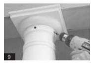
**9**. Place the capital on the shaft and pre-drill and countersink holes at an angle through the shaft into the capital. Install rust resistant screws to secure the shaft to the capital.
