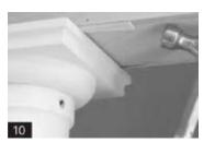
**10**. Be sure the shaft is centered under the soffit. Use shims to secure the capital in position under the soffit,
