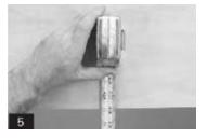
**5**. Measure the overall opening height. Subtract the height of the base and capital from the overall opening height to determine the shaft length.
