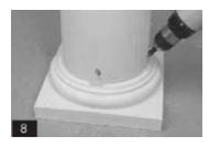
8. Pre-drill and countersink holes at an angle through the shaft into the base. Install rust resistant screws to secure the shaft to the base. Remove any excess silicone sealant.
