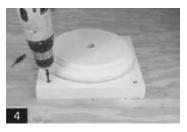
**4**. Pre-drill and countersink holes through the base and into the floor. Secure the base to the floor with rust resistant screws,
