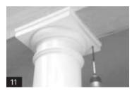
**11**. Pre-drill and countersink holes through the capital and into the soffit. Install rust resistant screws to secure the capital to the soffit.
