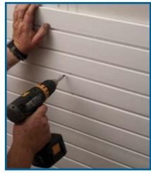
**STEP 5**: Proceed to the next slatwall panel, lining up the tongue on the bottom edge with the groove on the top edge of the previous panel. Repeat **STEPS 2-4** until all panels are installed.
