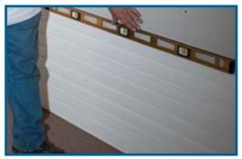
**STEP 4**: Screw the slatwall to the wall in the center of the slot at every wood stud along the top and bottom slats with #6 or #8 drywall flat head screw. Be careful not to over tighten the screws. Use self-tapping drywall screws over metal studs. Masonry wall should first be framed with wood studs.
