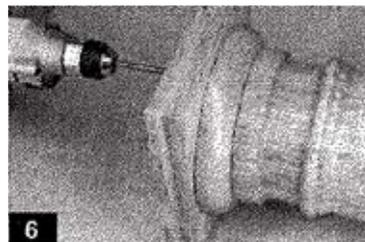
**6.** Attach the capital to the shaft by pre-drilling and countersinking holes through the capital into the top of the shaft. Make sure the edges of the base and capital are aligned. Secure with rust resistant screws.
