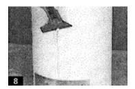
8. Allow the polyurethane adhesive to thoroughly cure and cut away the straps. Use a putty knife to remove any excess polyurethane adhesive. Use automotive body filler to cover any voids along each seam. Sand both seams smooth.
