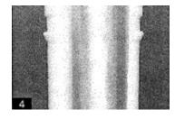
**4.** Align the column halves together around the structural support and join together.
