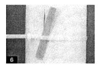
**6.** Larger diameter columns require joining two straps together. Temporary shims maybe required to align the column seam. The shims are removed after the polyurethane adhesive has cured.
