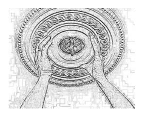
Once the medallion is cut, make sure the junction box is free and clear to work with. Make sure the wires and screw holes are accessible so that the fixture will fit nicely. Make sure the threaded bolt or nipple is long enough to reach from the junction box to the fixture once the medallion will be in place. If everything is fine then remove and get ready to glue it on.
