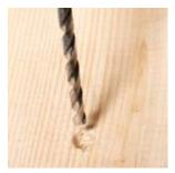
Drill a new hole approximately 1 to 1  $\mbox{\sc s}''$  deep using a  $\mbox{\sc s}_{16}''$  drill bit.
