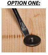
Remove the old metal insert with a screwdriver.
