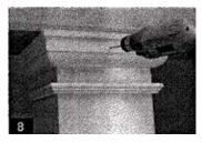
8. Slide the capital into place and pre-drill through the capital and shaft for screws or toggle bolts. Install rust resistant screws to secure the capital into place. Use automotive body filler to cover the screw heads and apply a bead of paintable silicone sealant at the joint between the shaft and capital.
