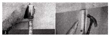
**2**. Measure the overall opening height. Raise the soffit slightly with a sturdy brace to allow positioning of the column during installation.
