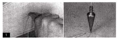
**1.** Drop a plumb bob from the center of the soffit to determine the column's center point on the floor. Mark this point for reference to align the column in the proper position under the soffit.
