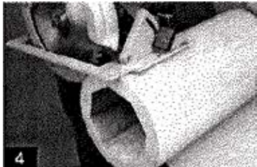
4. If trimming is necessary, trim from the base of the shaft. The load must be evenly distributed around the entire column circumference.
