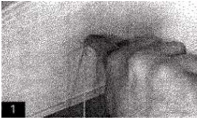
1. Drop a plumb bob from the center of the soffit to determine the column's center point on the floor. Mark this point for reference to align the column in the proper position under the soffit.
