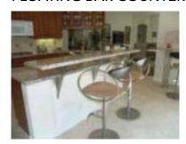
The floating bar countertop application is similar to the elevated bar countertop application in that the supported bar is elevated above a base countertop. However, this application differs from the elevated bar in that entire floating bar is supported entirely by the brackets.
