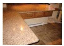
The cabinet supported countertop is the most common application used with countertops. When a countertop is supported by a cabinet island or row of cabinets the floor to counter structure of the cabinets gives the countertop the best possible support. In these applications it is unnecessary to support an overhang of under 4 inches (by cabinet industry standards).
