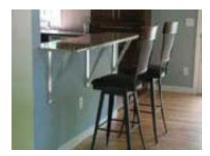
The elevated bar countertop is generally supported by a knee wall (also called pony wall or stud wall). The knee wall can be of varying heights but it is made out of 2 x 4 wood or metal studs and generally covered with sheetrock or paneling. The knee wall will extend a specified distance about a base countertop below and form a backsplash on the interior edge of your cabinet support countertops.
