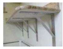
The wall mounted bar countertop is another application where the full weight of the counter is supported entirely on the brackets holding up the countertop. These types of mounts may also be called shelves or mantles.
