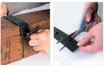
Lay the strap along the beam. Make sure that the straps three bolt heads are even on the top of the beam.
