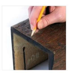
Draw a light pencil line perpendicular to the center of the beam strap.
