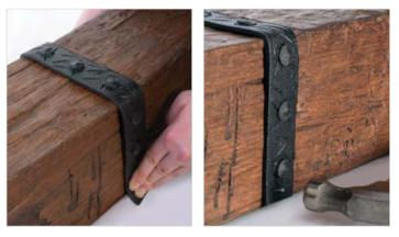
Align the center of the strap with the marks made in Step 1. Press firmly on the strap working from the center up each side to ensure good contact between the adhesive and the beam.
