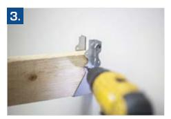
Lightly push the lumber into the joist hanger. This structure will support your beam. Secure the lumber with screws.
