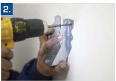
Use screws to fasten a joist hanger to the wall
