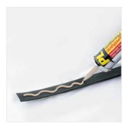
Apply a bead of adhesive to the back of the strap.
