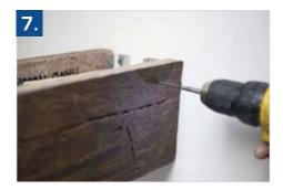
Screw the beam to the support structure. For the best result, use screws with small heads (trim head screws).
