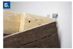
Slide your beam onto the support structure. The beam should fit perfectly.
