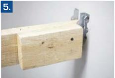
Screw wood blocks on the support structure.
