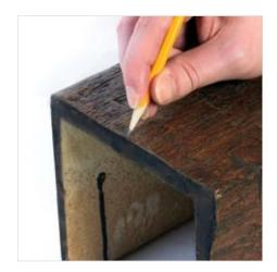
Draw a light pencil line perpendicular to the center of the beam strap.
