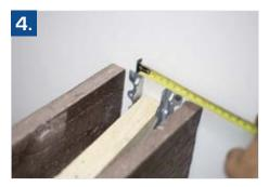
The beam has to fit perfectly, if not, you will need to fill the extra space with wood. Measure the negative space. This will show you how thick it has to be.
