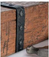
Align the center of the strap with the marks made in Step 1. Press firmly on the strap working from the center up each side to ensure good contact between the adhesive and the beam.
